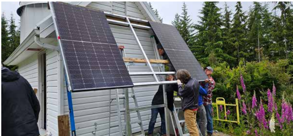
Installing the solar panels at the VRO
