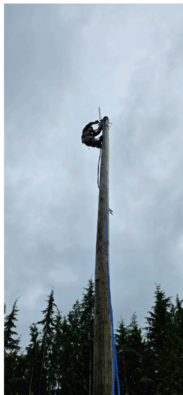
Alan Jones climbs a pole to remove decommissioned electrical wire
