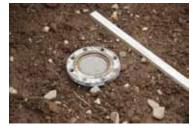
Here you can see the flange more clearly. It has 8 mounting holes of which I used 4. These holes are sized for 3/4" bolting, much stronger and stiffer than the 1/2" called for by the commercial plans.
