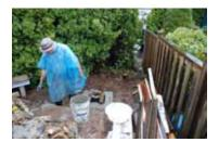
Of course it has to rain when the concrete work has to be done. You can see the top of the lower pier with the flange. It is being supported by a couple of 2 x 4's while I pour the concrete that I am mixing in the Rona pail.
