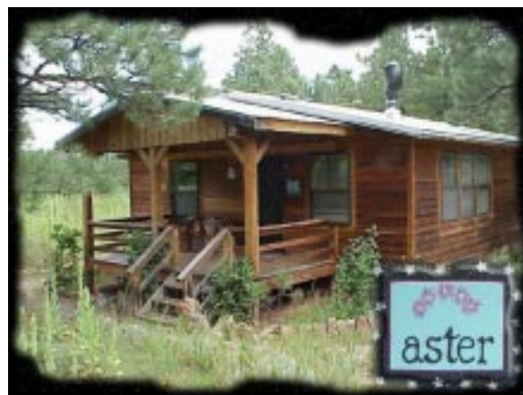
Exterior of Aster Cottage at the Star Hill Inn, northern NM Rocky Mountains
